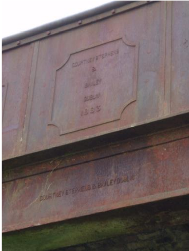
Plate 8: Detail of Osberstown railway bridge
