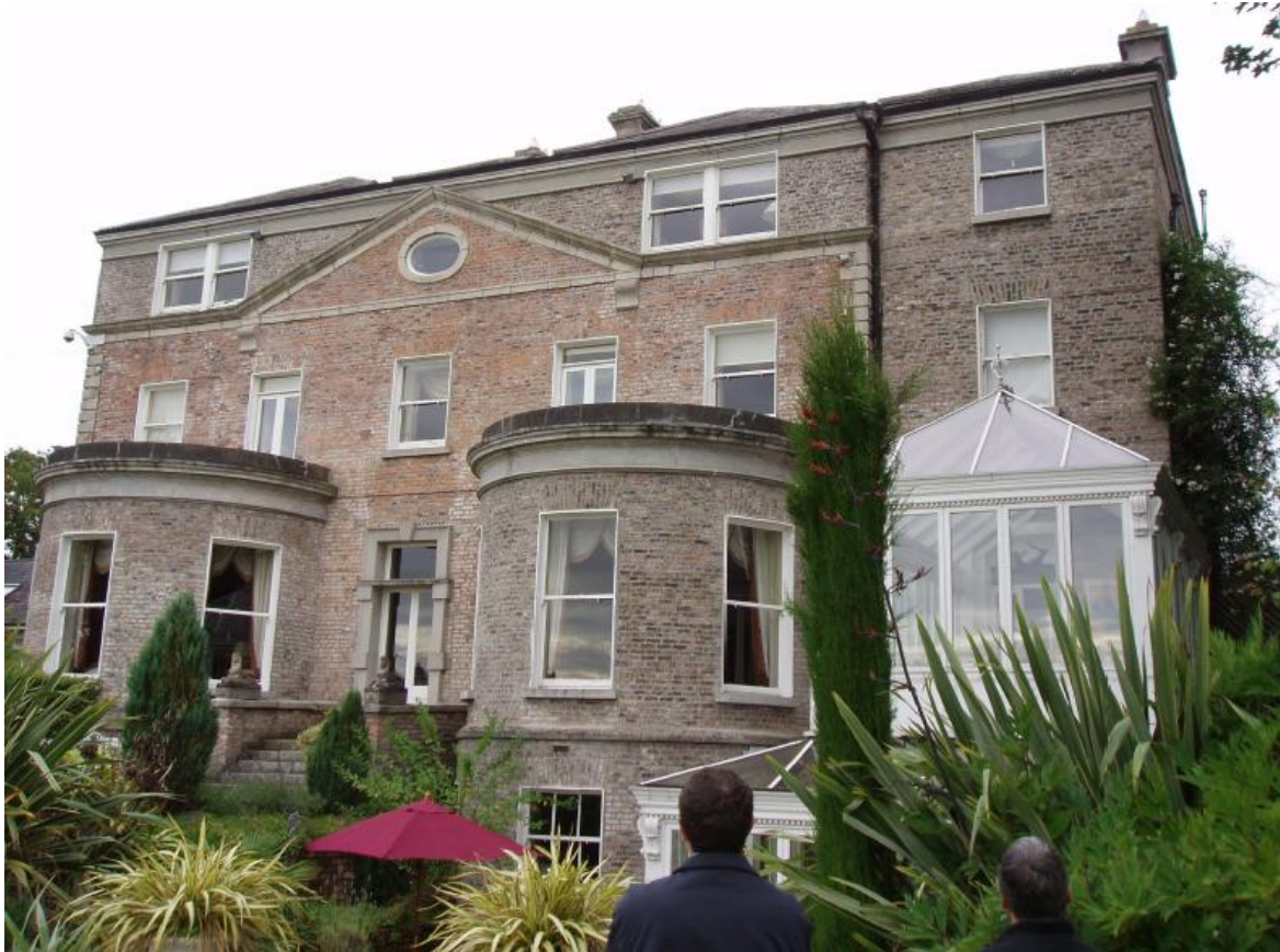
Plate 1: Osberstown House, east elevation (Gifford Ref 158/163)
