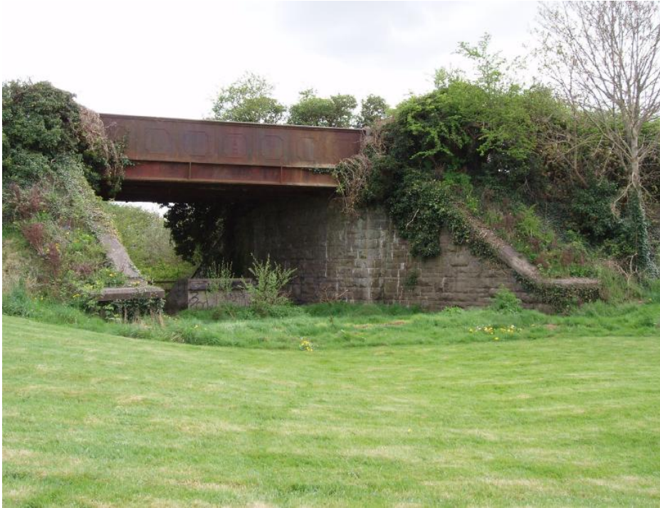
Plate 7: Osberstown railway bridge (Gifford Ref 160)
